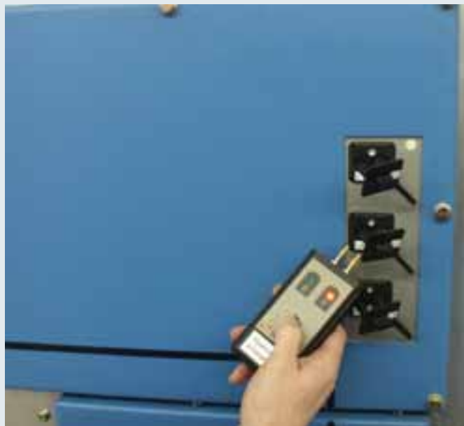
Self-test of the DEHNcap/A voltage indicator.
