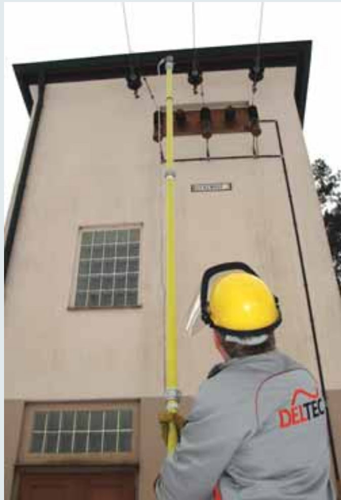
Earthing rod consisting of a top section, intermediate section and sealing unit.
