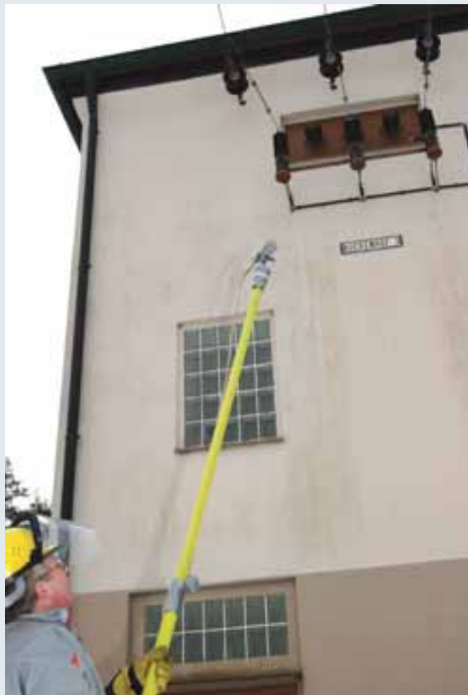
Telescopic earthing rod with aluminium cone coupling and phase screw clamp
