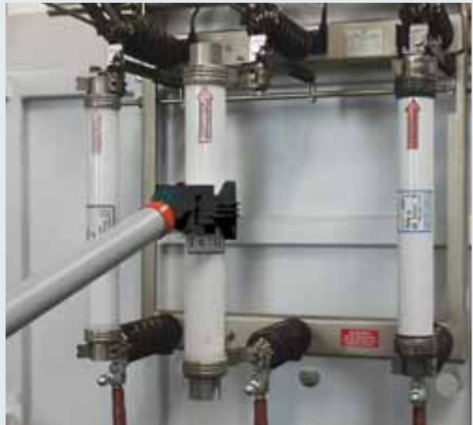
Angled (20°) SZ fuse tongs for inserting and removing h.v.h.b.c. fuses.
