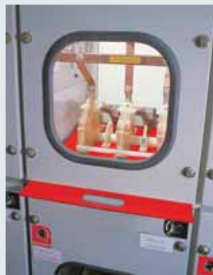
Inserting an insulating protective shutter, type A4.
