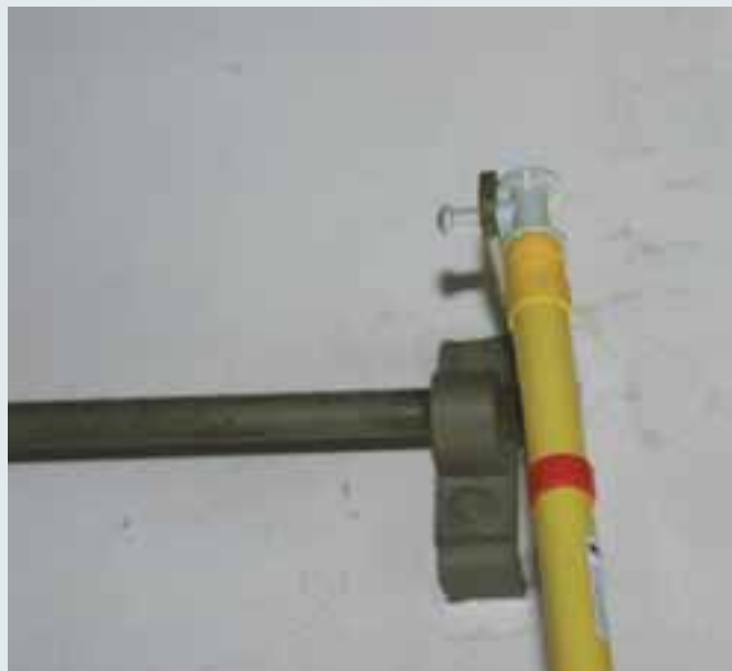
Switching a disconnector by means of an IS SK insulating rod with switching rod head.
