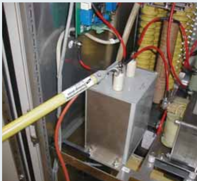
Single-pole device for discharging static charges.
