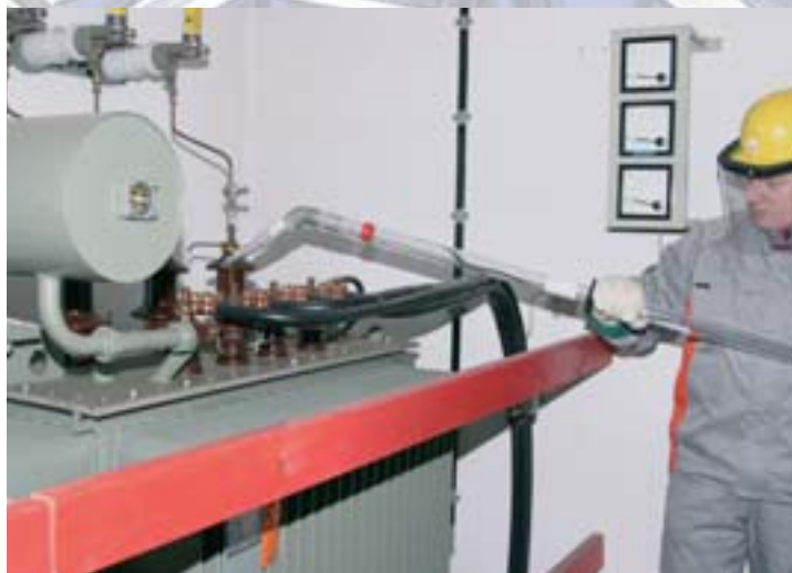
Safe cleaning under live conditions with DEHN equipment!
