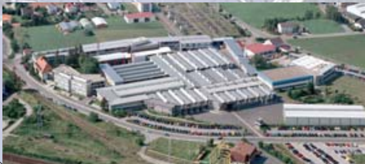
Centre of lightning and surge protection and safety.
